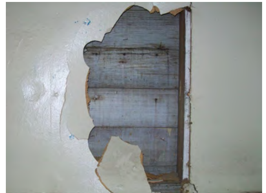
Above- One of the numerous holes in the walls at the Field House.
